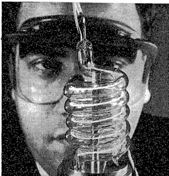
**SUPER LIGHT SOURCE:** Dr. Theodore H. Maiman of Hughes Aircraft Company, Culver City, Calif., studies new electronic device called a laser. A light source surrounds a rod of synthetic ruby crystal that, when properly activated, can generate a "coherent" beam of light brighter than that emitted by the center of the sun.
